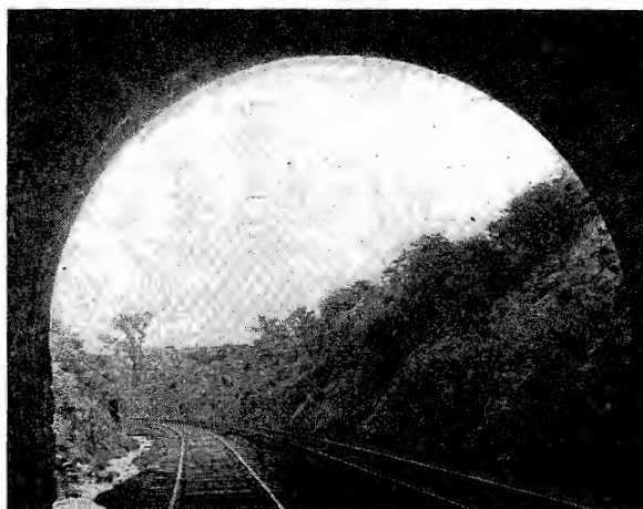
Overhead catenaries or cross wires supporting the v-h-f redistribution antenna, as seen from the west end of the Mt. Airy Tunnel. Wire runs out of the tunnel roughly paralleling the tracks for a short distance.
