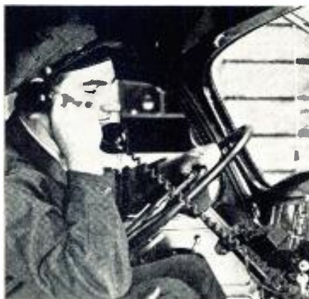
W.E. f-m telephone service system, installed by Bell System.
