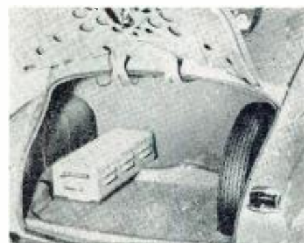
(Left) Federal transmitter-receiver unit, in taxi trunk compartment.
