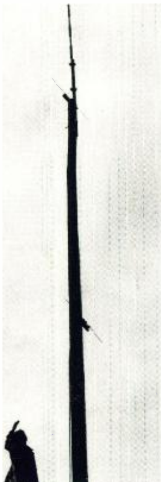
Two horizontal-polarized dipoles and triple skirt antenna at the central station doghouse on Selden Hill.
