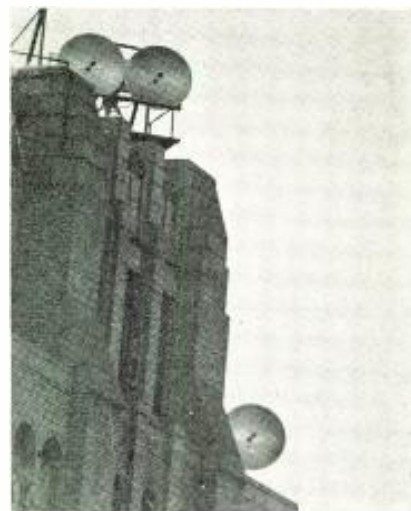
Western Union microwave relay reflectors at the Philadelphia terminus for handling communication and television channels. (Courtesy Western Union Telegraph).
