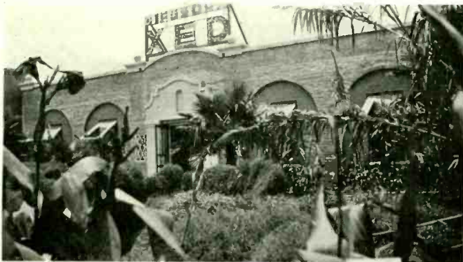
The main building of the station, then XED (November, 1933).
