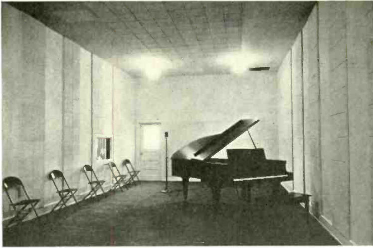
VIEW OF MAIN STUDIO FROM RECEPTION ROOM.
