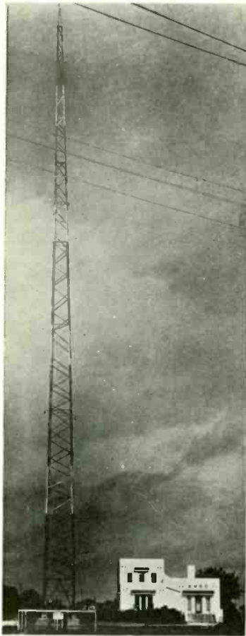
THE LEHIGH VERTICAL RADIATOR OF KVSQ, ARDMORE, OKLAHOMA.
