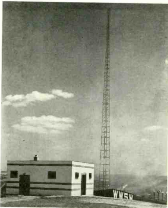
THE NEW 154-FOOT, TYPE CK, BLAW-KNOX VERTICAL RADIATOR OF RADIO STATION WWSW, PITTSBURGH, PA.
