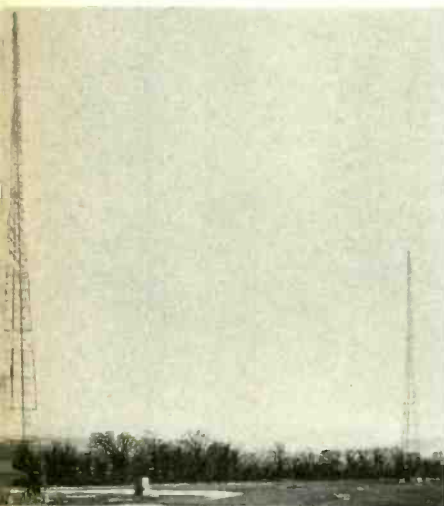
WSYR'S (SYRACUSE, N. Y.) DIRECTIONAL ANTENNA SYSTEM. EACH OF THESE IDECO SELF-SUPPORTING VERTICAL RADIATORS ARE 330 FEET HIGH.
