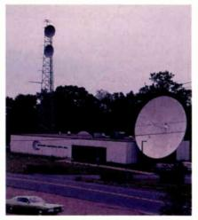
Greater Hartford Cable TV, August 1979: Notice the 10-meter antenna pointed at Satcom 1, the only satellite needed at the time.
