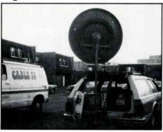
These pictures were taken to prove that the antenna cleared the buildings and trees in front, when receiving Satcom 3-R, as well as to pinpoint the exact dish location for the proposed small earth station.
