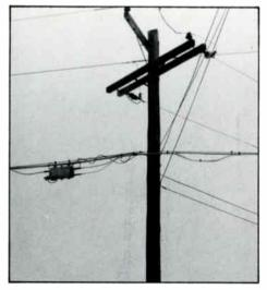
That's a directional tap on the left side of the amplifier. Can you imagine trying to install a pay service trap on the port of that tap using a line belt and hooks?
