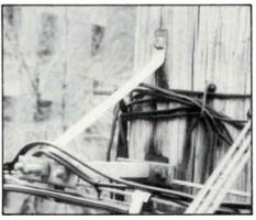
The straight extension bracket is used to maintain clearance over streets or to add a second cable when clearance is a problem.
