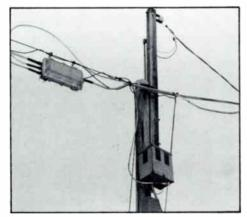
What is wrong with this picture? Nearly everything! Out of the picture to the left is a directional tap. A ladder placed between amplifier and pole will crush the drop cable. The loose power cable is asking for a sheath break, as is the looped feeder. Now how would you climb this pole? At least it has a power cutout switch.
