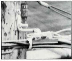
The T-Alley bracket is used for alleys or building junction poles.
