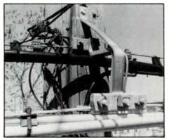
The CATV L Bracket is used on the majority of poles to facilitate makeready.
