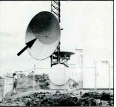
A typical microwave antenna (note the arrow pointing to the feedhorn).
