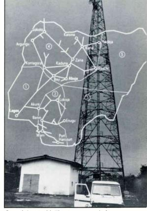
One of the steel lattice towers erected in Nigeria that carry the antennas via which television, telephone and telex signals are transmitted.
