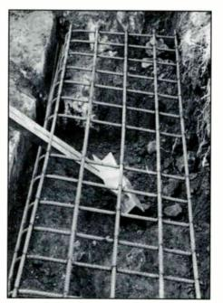
eter vertical shafts. Guyed tower foundations usually consist of a pier and pad base for the tower and three or more ''dead-man'' buried anchor blocks.
