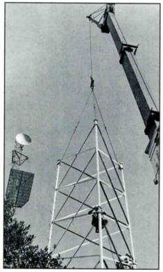
Clockwise from above: self-supporting tower being erected using a crane; pier-andpad foundation for guyed tower base under construction; foundation reinforcements for ''dead-man'' anchor block for guyed tower,
