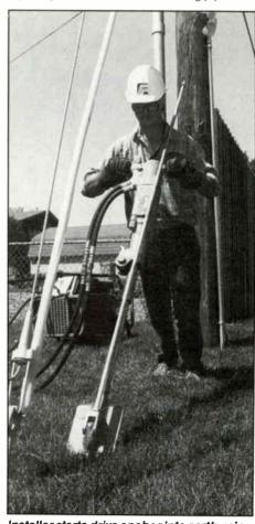
Installer starts drive anchor into earth using standard jackhammer and drive gad.
