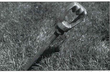
After the load locker is removed, the thimble is screwed onto the end of the anchor rod, ready for guying.
