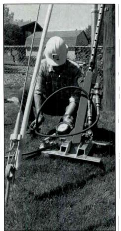
With a power source, the load locker pulls up on the anchor rod, rotating the anchor into load lock position to the desired holding capacity.
