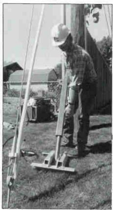
A tubular setting pipe is screwed onto the end of the anchor rod. The load locker base and hydraulic ram are then put in place over the pipe.
