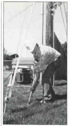
After the anchor is all the way in the ground to the desired depth and angle, the drive gad is pulled out of the ground.
