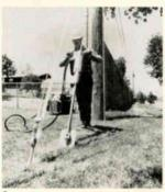
One man at ground level drives Manta Ray with jack hammer.
