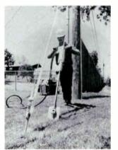
One man at ground level drives Manta Ray with jack hammer.
