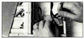
Step 14: Wrench tighten the cable's F connector.
