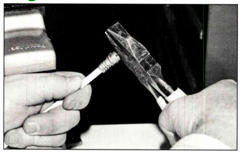
The video portion in interactive training shows the student how to perform tasks like installing an F connector.
