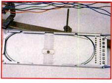
Step 4: Remove the tube from the optical fiber strands. Using a dry towel, wipe the excess gel from the fibers then attach the tube to the splice organizer tray. Most closures accomodate between 36-48 inches of excess tube length. The additional 48-60 inches of fiber should be wrapped neatly in the organizer tray.
