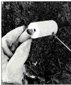
**Photo 7:** Tap the starting material out of the weld metal container into the hole in the center of the mold cover.
