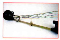
Step 3: Secure the two cable ends into the closure to provide the required strain relief. Optical cables are designed with components called strength members to give support and carry loading. These are typically steel wires, fiberglass-reinforced plastics and aramid yarns such as Keylar.
