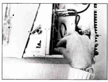
Step 7: Install the new connector from the front and replace the nut.
