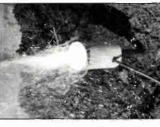
**Photo 8:** Ignite the starting material with the flint ignitor, holding it one or two inches from the hole in the mold cover.
