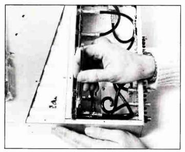
Step 5: Remove the nut from the chassis connector.
