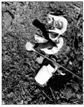
**Photo 9:** After 30 seconds to a minute, the mold may be broken off the finished Cadweld.
