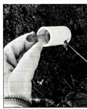
**Photo 5:** Pour the weld metal into the mold. Note that a separate starting material will remain in the bottom of the weld metal container.
