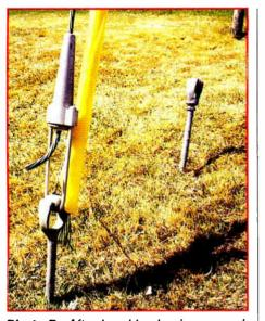
**Photo 7:** After Load Locker is removed, thimble is screwed onto end of anchor rod, ready for guying.
