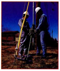
**Photo 5:** Adapter setting bar is screwed onto end of anchor rod. Load Locker base and hydraulic ram system are placed over the adapter setting bar.
