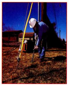
**Photo 3:** Installer pulls drive gad out of ground.
