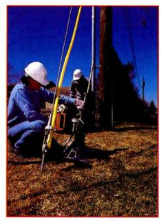
**Photo 6:** Power source operates Load Locker, pulls up on adapter setting bar, rotating anchor into position, to the desired capacity as indicated by the gauge on the Load Locker.
