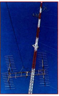
A stagger stacked quad-array lifted in the air.
