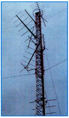
The tower can be protected by installing a dissipation array on the top, and a dissipator set on each top-mounted DC ground antenna.
