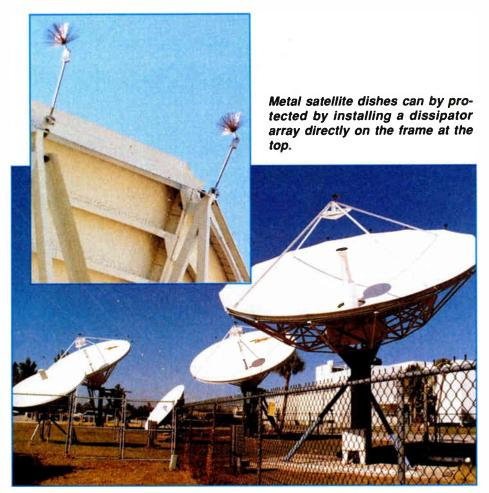
in 500 feet or so of the ground, the electric field intensity on the ground becomes so strong that objects and structures on the ground begin to break down electrically and respond by shooting off streamers up toward the stepped leaders. When a streamer connects with a stepped leader, the ionized path becomes the channel for the main lightning discharge. The other streamers and stepped leaders never mature.
