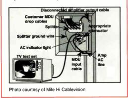
c) Does not reconnect the output cable.
