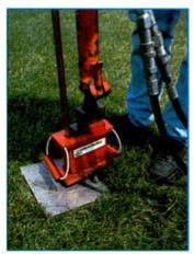
Photo 5: The ground rod is driven into the soil until the Sidewinder reaches ground level and contacts the release plate.
