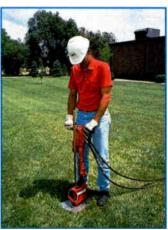
Photo 8: As before, the rod is driven into the soil until the Sidewinder again reached ground level and contacts the release plate.
