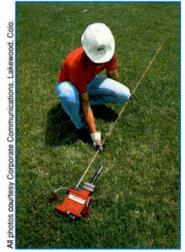
Photo 1: The ground rod is inserted into the Side-winder's jaws.
