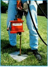
Photo 9: Steps 6 through 8 are repeated as necessary until about 1 foot of the rod remains above the ground. The Side-winder is then placed on the top of the rod for the final step.
