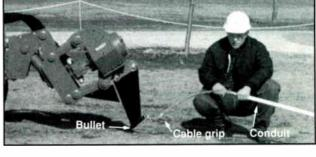
**Figure 3:** Plowing in cable with a vibratory feed (chute) plow
