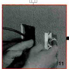
wall, following the penciled outline (Photo 8). He continues by removing the two bottom half-inch knockouts from the 4-inch square box and discards them (Photo 9). He also installs a half-inch threaded chase nipple, which provides a smooth surface for the drop's installation and any future movement (Photo 10). He then installs a half-inch lock ring to secure the chase nipple to the 4-inch square box that accompanies both chase nipple ends with an insulating bushing (Photo 11).
