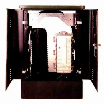
Fiber Storage Bracket is capable of storing up to 300 feet of Fiber Optic Cable.
