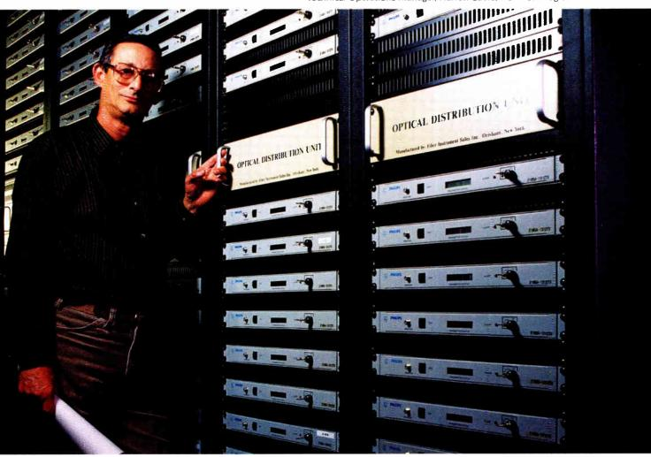
"Every quarter we test our fiber optic COAX system and compare current trace signatures to the originals to spot problems before our subs view them. We're shooting Laser Precision's mainframe and Mini-OTDRs, which let us pinpoint faults, too.
