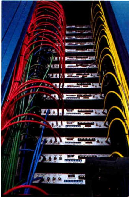
**Precision video cable (above) runs of up to 100 feet connect a wide variety of rack-mounted broadcast equipment.**
