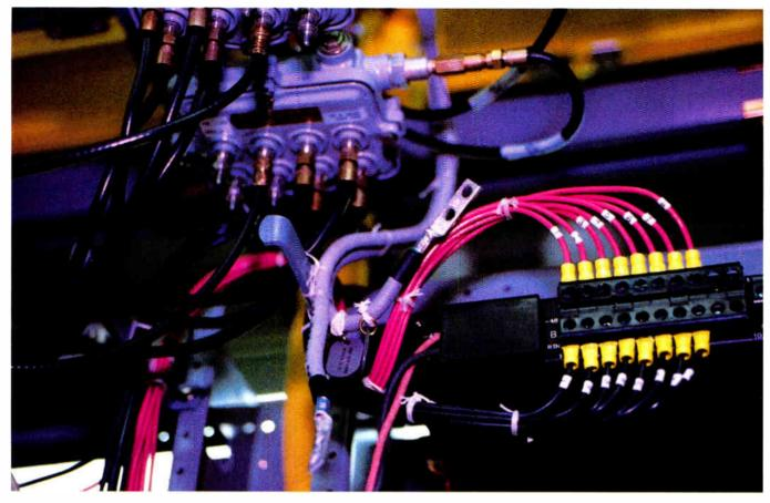
Video feeds to the 1,550 nm transmitters that lead to MediaOne's 41 distribution hubs.
