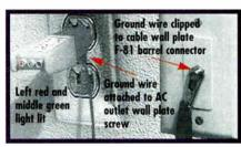
Figure 2: Temporarily grounding ungrounded polarized two-slot receptacle
