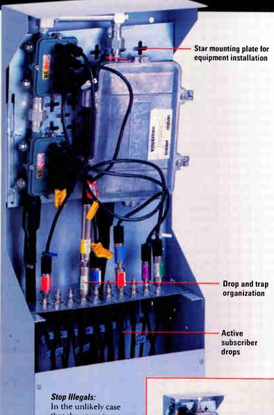
In the unlikely case that the cover is ever forced off, there still remains a second line of defense which prevents an illegal hook-up because all of the unconnected drops are still hidden and protected in the lower inner box.
