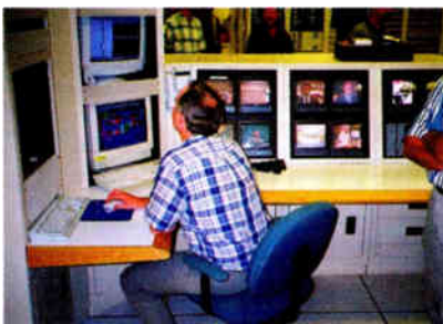
MediaOne's Western Regional NOC
