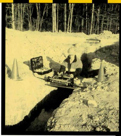
When choosing a splicer, be sure to evaluate its field loss, which indicates expected performance under actual field conditions, allowing for variations in climate, cleanliness, cleaving and operator training. Both photos are courtesy of Siecor.
