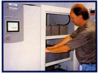
Battery-powered universal power supplies, such as this 50 kW unit, provide temporary electricity to Cable TV Mongtomery's headend until the onsite generator turns on.
