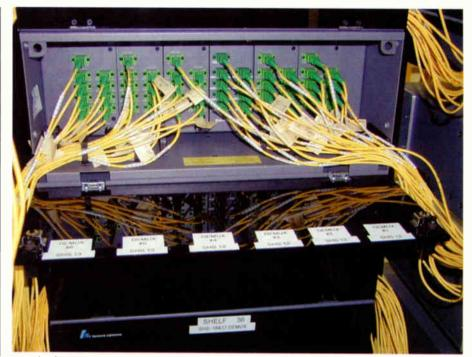
A rack of  $1 \times 8$  passive optical multiplexers and demultiplexers at an AT&T B&IS primary hub for its Aurora, Colo, system. Photo courtesy of Harmonic Inc.
