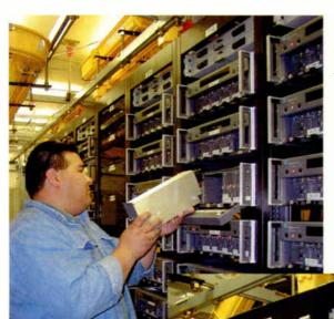
In another look at the AT&T B&IS Aurora system, at left, a technician mounts a narrowcast forward path transmitter module. Below, the tech tests the RF signal level on a return path receiver. Both photos courtesy of Harmonic Inc.
