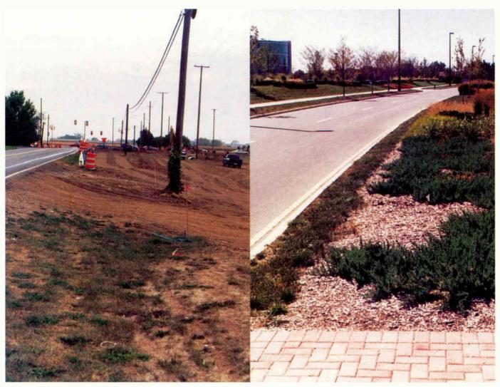
DubLink in action: At left, DubLink crews work right along with road construction crews widening Rings Road in Dublin, Ohio. The municipality is installing its own telecommunications infrastructure, on which providers can lease space. The arrangement is designed to prevent having the city's landscaped rights of way, such as the one at right along Emerald Parkway, continually dug up for new telecommunications construction.
