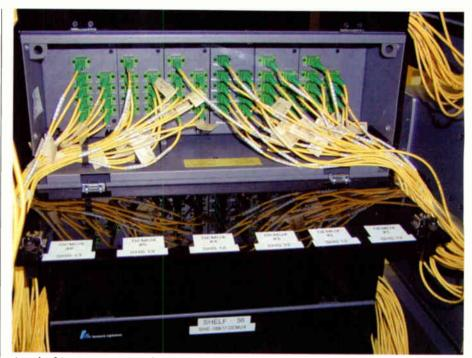
A rack of 1 x 8 passive optical multiplexers and demultiplexers at an AT&T B&IS primary hub for its Aurora, Colo, system. Photo courtesy of Harmonic Inc.
