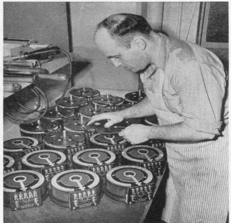
The Duratrak process, which follows baking, coats the brush track with the silver surface shown on these partially assembled units.
