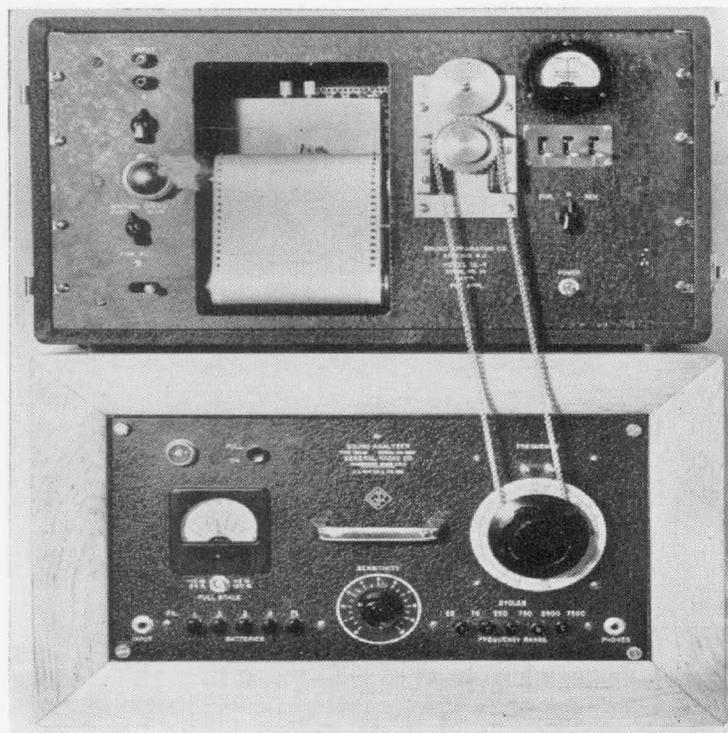
Figure 2. The recorder coupled to the General Radio Type 760-B Sound Analyzer.
