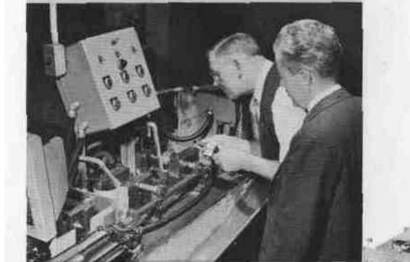
This machine, designed and built at General Radio, automatically mills from blocks of aluminum complete rotors and stators for variable capacitors.
