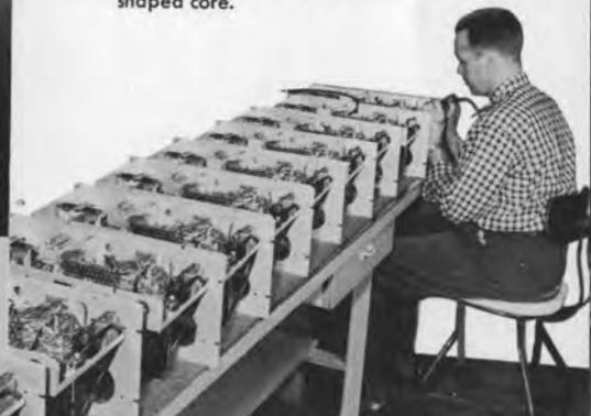
In the assembly department, each man assembles a group of instruments, performing operations on each successively. Versatility is a prime requirement, because in the course of a year a man will assemble dozens of different products.
