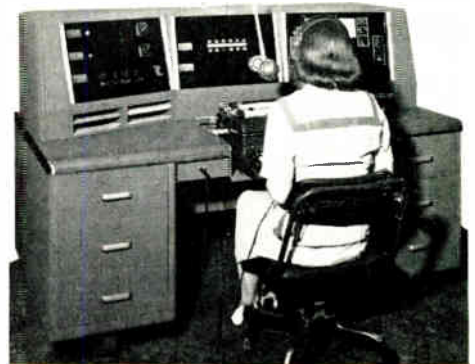
Control console installed by National Airlines at La Guardia Field.
