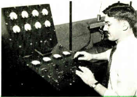
Section Chief G. R. White measuring the conversion transconductance of a mixer tube on a Bendix-built bridge.
