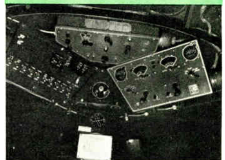
Overhead control box, center, and ADF control panel, right, installed in DC-3.
