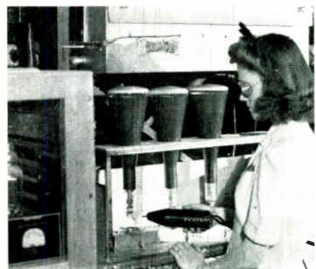
When tubes are partially exhausted, operator applies spark coil test to the tube. Color of resulting glow reveals leaks.
