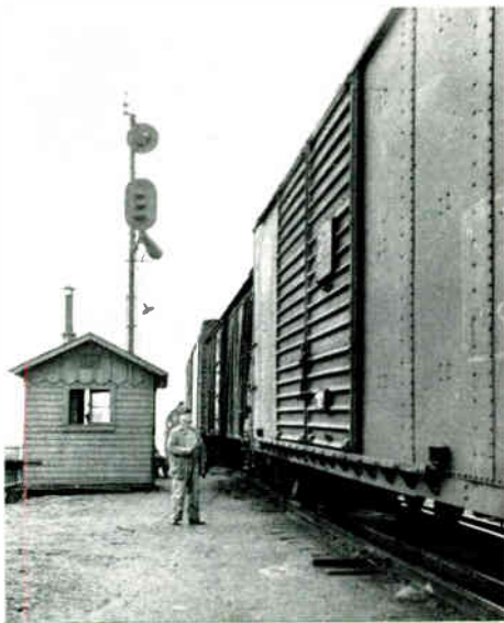
Figure 4—MS-101A ground plane antenna atop signal pole at one of the B & O fixed stations.
