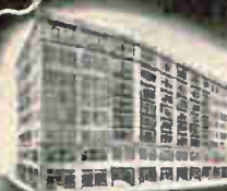
C-D WORCESTER, MASS., PLANT
