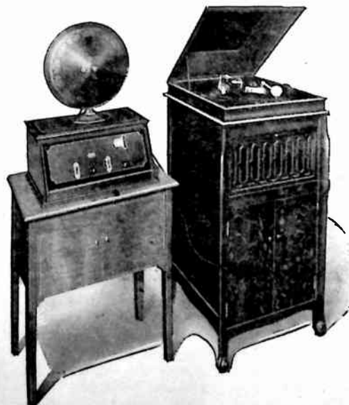
This picture shows how the Merola takes the place of the tone arm of the phonograph and how it is attached to the radio.
