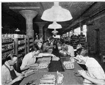
Assembling Tuning Condensers
