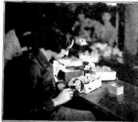
3.—The title of this picture is "Assembling the Condenser Gang." But it has no reference to the underworld. It means that the stator assemblies are put into "bathtubs," the rotor assemblies are mounted on the rotor shaft, then the pinion bracket is mounted, next the pinion and the dial.
