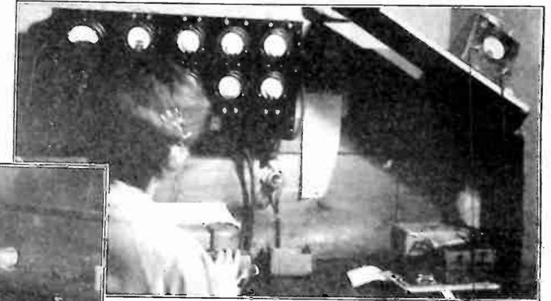
8.—Power Converter Test. In this sound-proof testing room, the young lady tests the power converter chassis. She also tests the power transformer, tests to see if unit is in working condition, inserts tubes to see if each tube will get the proper voltage, and finally, she tests for mechanical hum in the transformer.
