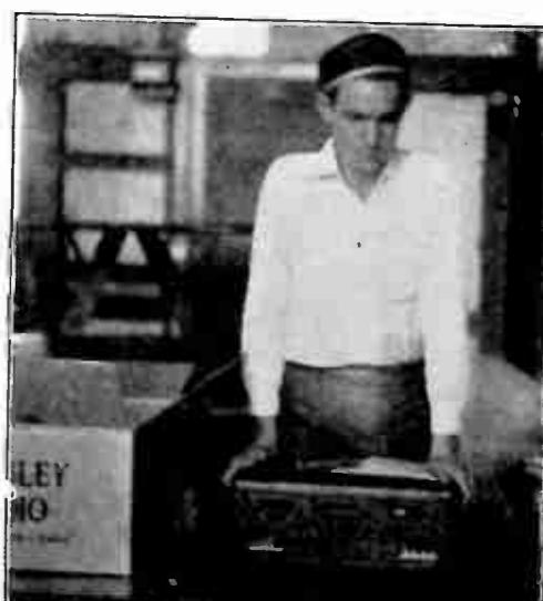
12.—The Packing Line finds the Showbox almost ready to leave the plant, right. The finished sets travel down a belt and go through the various processes of shipping, which include tagging, putting instructions into each set, etc. Here the man is about to place a Showbox in a strong shipping carton.
