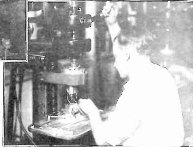
2.—Tapping. After the rotor and stator assemblies have been trimmed on a punch press, the holes are tapped, 2 holes at a time. This means they are threaded so that screws can be put in.
