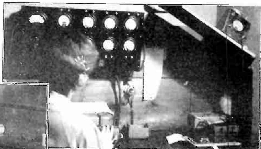
8.—Power Converter Test. In this sound-proof testing room, the young lady tests the power converter chassis. She also tests the power transformer, tests to see if unit is in working condition, inserts tubes to see if each tube will get the proper voltage, and finally, she tests for mechanical hum in the transformer.
