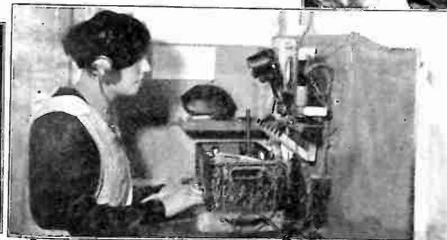
11.—More tests! The Showbox has traveled into another series of sound-proof booths and is thoroughly tested. If the handling has disturbed any of the parts or connections, it is discovered here. The set is balanced, tested to make certain it will cover the wave length or broadcast band, and checked for volume control.
