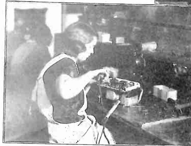
7.—The receiver travels on the chain conveyor to the Power Converter Department. The girl of the picture is soldering connections on the filter strips. The small meter hanging from the rack, is for testing open circuits on filter strips, before the set goes into the testing booth.
