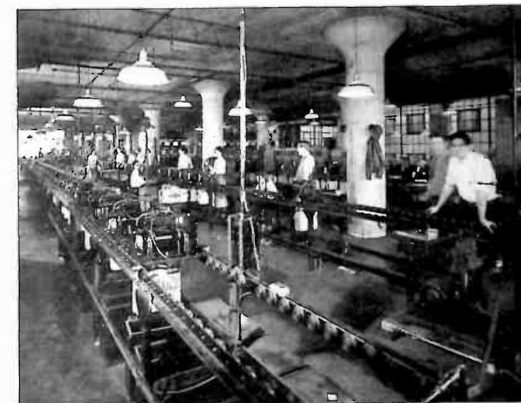
Section of the final assembly line for refrigerator units in the Crosley factory. Production facilities for Crosley Shelvadors
