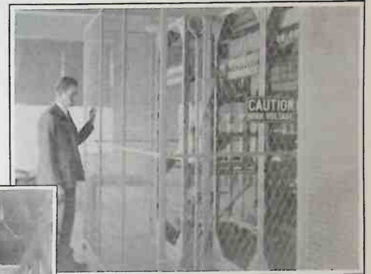
WHETHER YOU BELIEVE IN SIGNS OR NOT—You can't hurt yourself at WLW. To get inside the screen you must turn a lock which not only automatically shuts off the power but discharges the high-voltage condensers as well.
