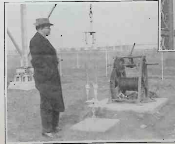
FOOD FOR THOUGHT—These insulators anchor the antenna lift cable. The gentleman has just touched the wrong end of them and has been both shocked and surprised. In the background is the hoisting tackle.
