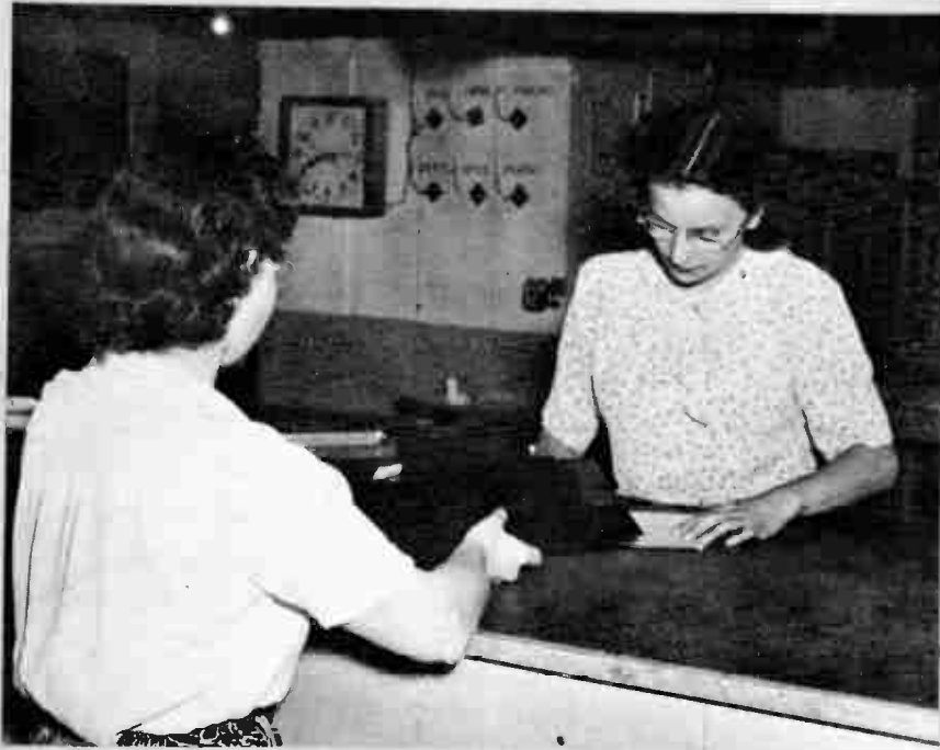
The beginning of the producing. An operator from the Punch Press department gets some tantalum sheets from the Materials Control Stockroom, and the manufacture will soon get underway
