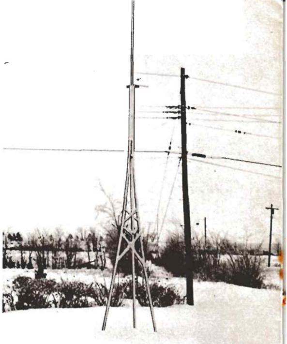
HANDY ANDY TOWER installed in snowy W2-land. If 22-foot long  $2 \times 4$ -inch lumber is substituted for the  $2 \times 2$ -inch lumber used on this model, over-all heights of 40 feet are possible.
