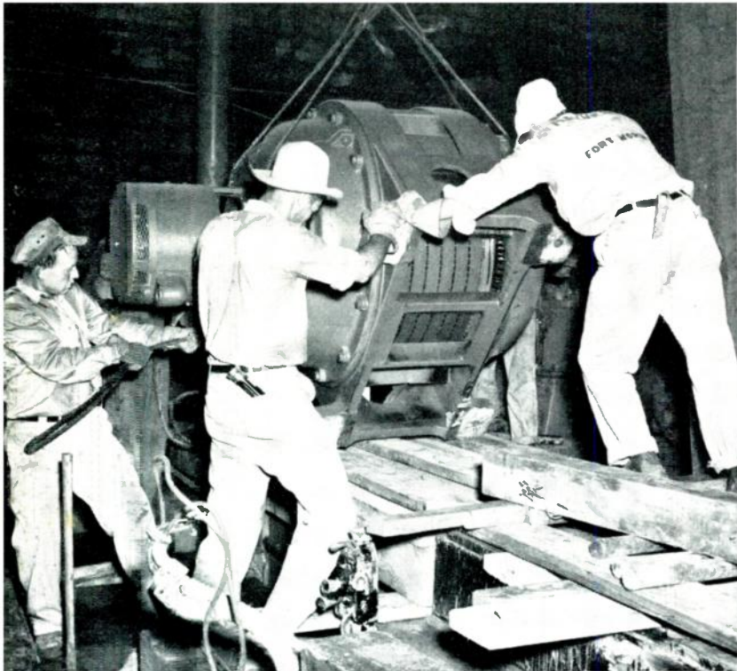
After rush shipment by special truck with police escort from Indiana to Texas, this 900-hp motor is lowered to its base at a flooded Fort Worth pumping station.
