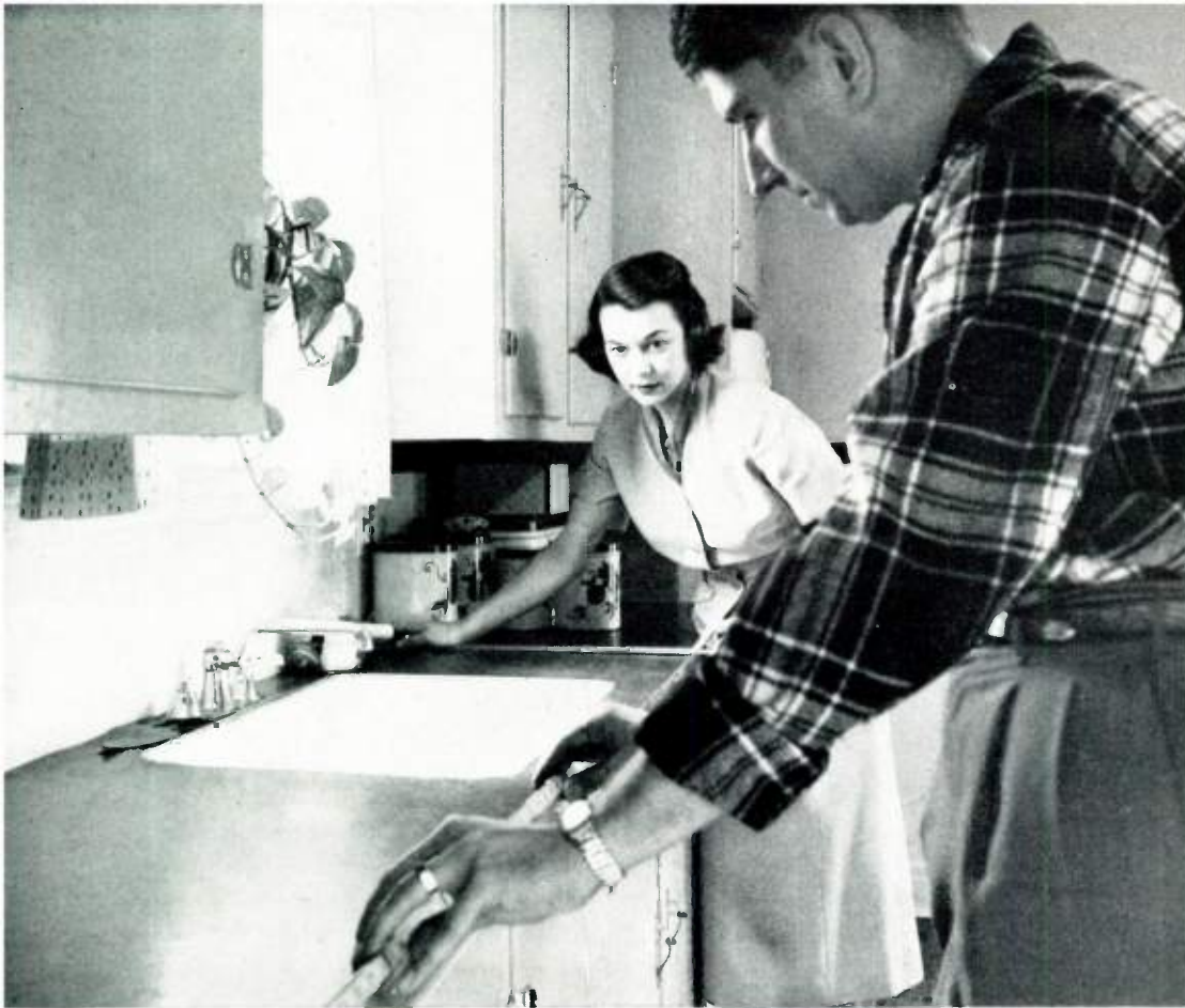
Starting at one o'clock Ard and Bess make their measurements for the first cuts. They allow \frac{1}{4} inch so the sheeting can be filed to exact size. The clocks below tell the time sequence of all important operations.
