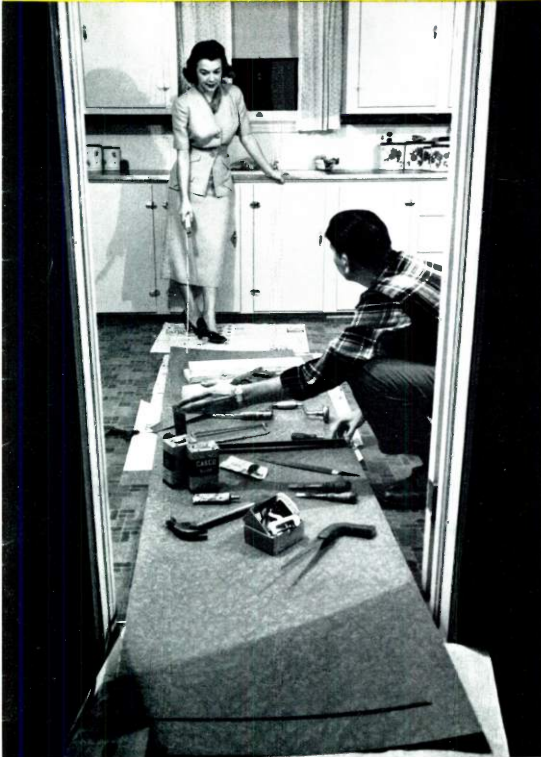
Checking his tool box, Ard finds everything he will use in resurfacing his kitchen counter. He has chosen decorative pattern Red Pearl. The sheets have come from the distributor cut to approximate counter size.
