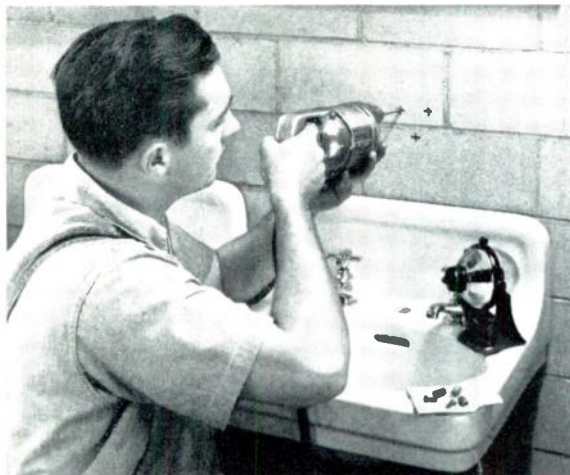
After more than a year of routine laboratory tests, the Carboly Department's "Live-Spiral" masonry drills were put in the field. Chicago was selected for the tests because construction firms there use a coarse, washed stone as aggregate in mixed concrete, a condition which gave rise to early customer complaints. The material was tough and hard to drill and could either make or break the drills, which are an adaptation of coiled spring and cemented tungsten carbide tips on ordinary steel masonry drills. Difficult construction jobs were selected in the area and Carboly supplied "Live-Spiral" drills to contractors on a no-charge basis. G-E engineers teamed with contractors' laborers to carry out the tests.
