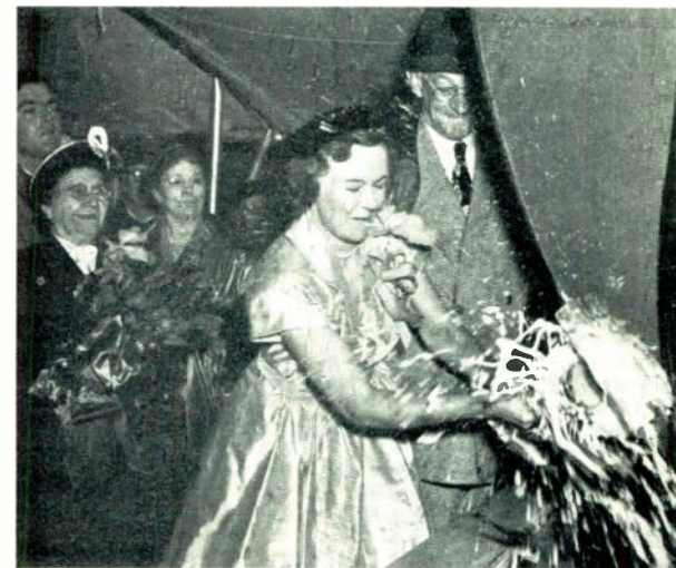
A submarine makes its first public appearance when it is christened and launched. At launching time the submarine is three-quarters complete.
