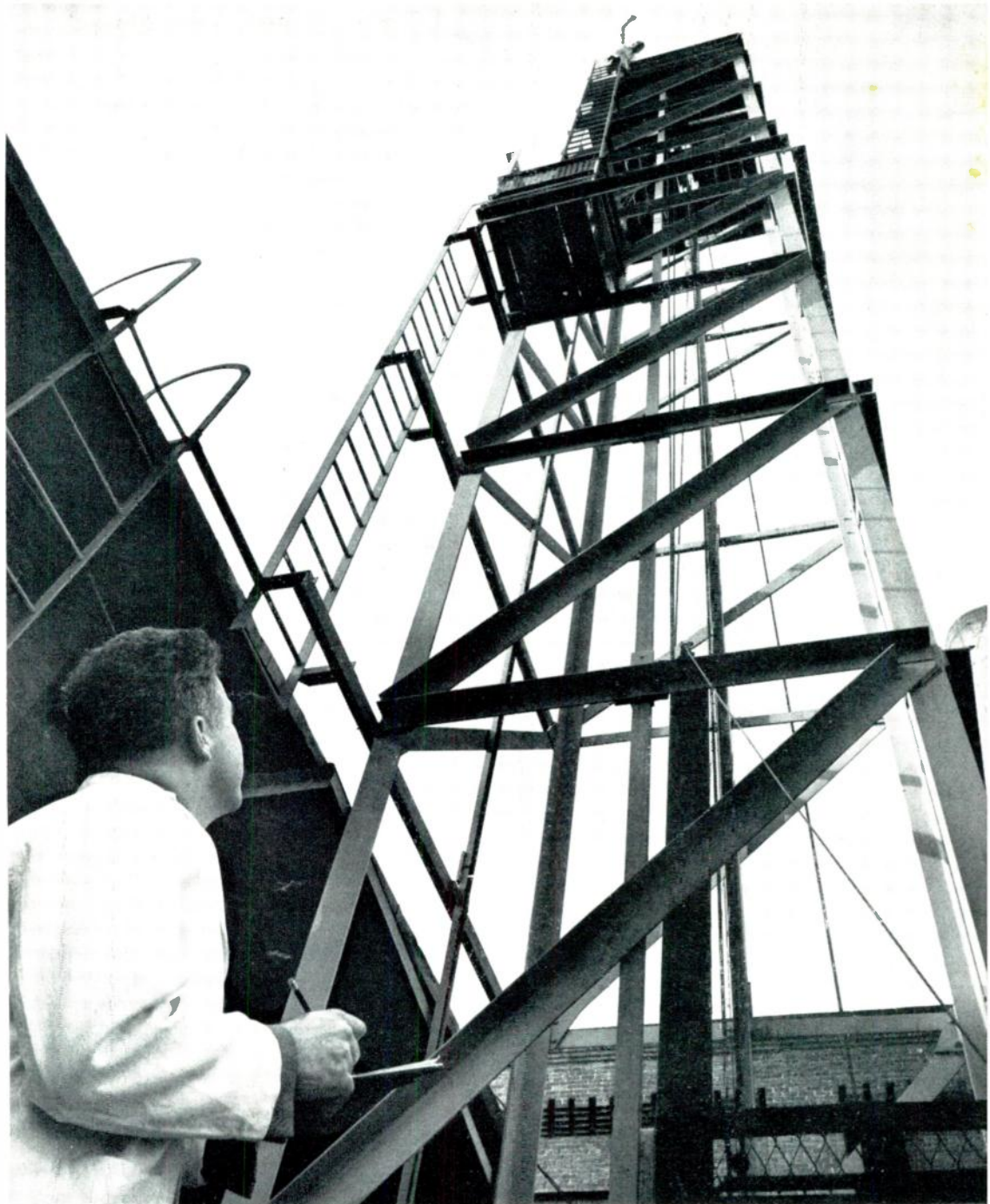
B. F. Roberts signals to W. K. McNitt from the top of the 85-foot tower at the Control Engineering Laboratory in Schenectady. The tower, built to test crane hoist equipment under actual working conditions, has a 70-foot free lift and a test load weight which can be handled in increments from a quarter ton to 22½ tons. All operating characteristics can be readily studied. The brake used on the hoist is of two-shoe, two-magnet construction designed three years ago and tested on the tower in a few days. Equivalent field tests would have required weeks. At full-speed lowering, a 15-ton load can be stopped in 1½ seconds. A 20-ton truck, traveling at 50 miles per hour, requires a distance of 110 feet to stop.
